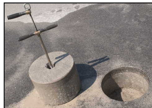
Central pilot hole aids in core extraction
