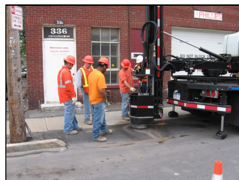
Proper horizontal and vertical alignment are important steps during set up
