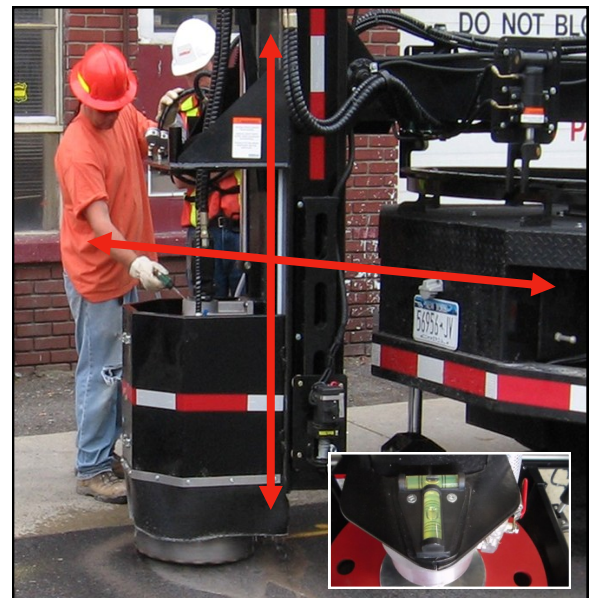
The coring drum needs to be set perpendicular to the horizon not the roadway.
