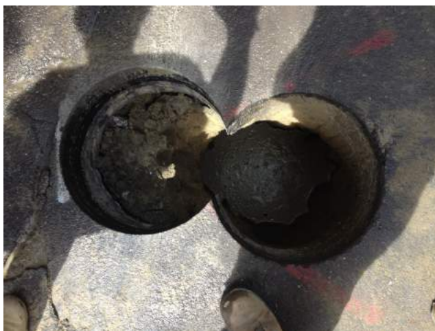
Two 18" diameter cores are cut to allow for greater access to buried facility
